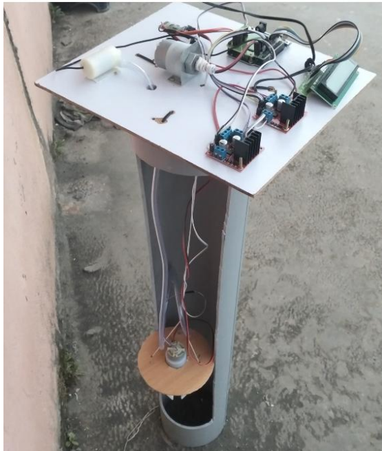
FIG 2: Hardware Implementation of prototype
