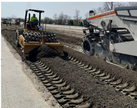
Figure 6. Flexible Pavement over Stabilized Subgrade
